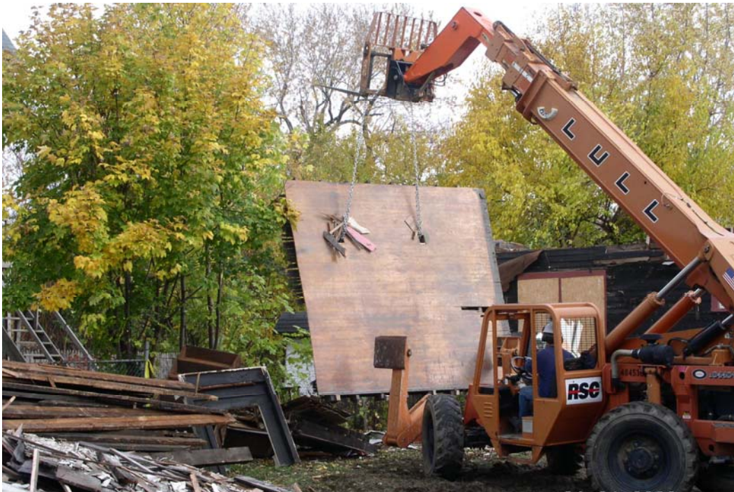
Photo 4 – Cleveland Deconstruction Initiative – Floor Removal
