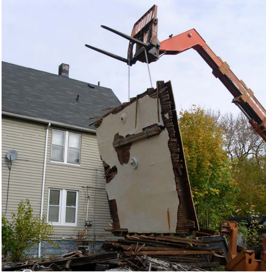
Photo 5 – Cleveland Deconstruction Initiative – Wall Removal
