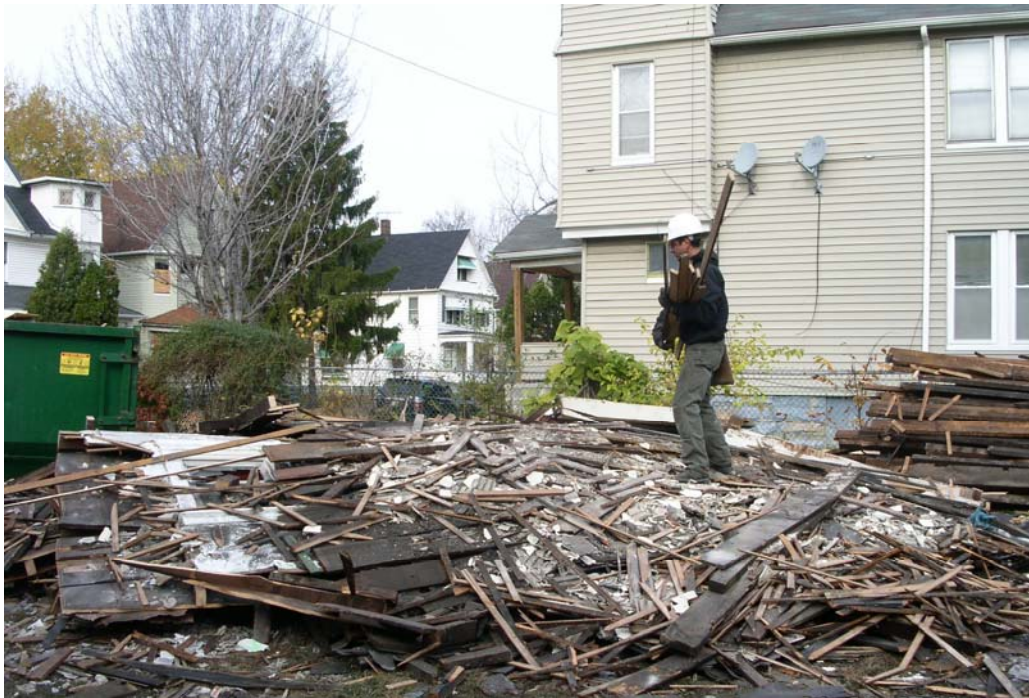
Photo 8 – Cleveland Deconstruction Initiative – Hand Dismantling
